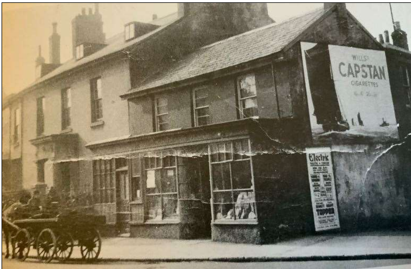
The row of terraced houses and a shop on South Street which were demolished to make way for the new police station. (Image courtesy of Paul Martin)
